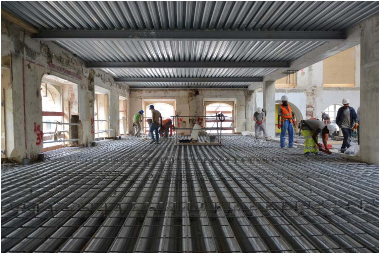
2 place Vendôme, renforcement de plancher
