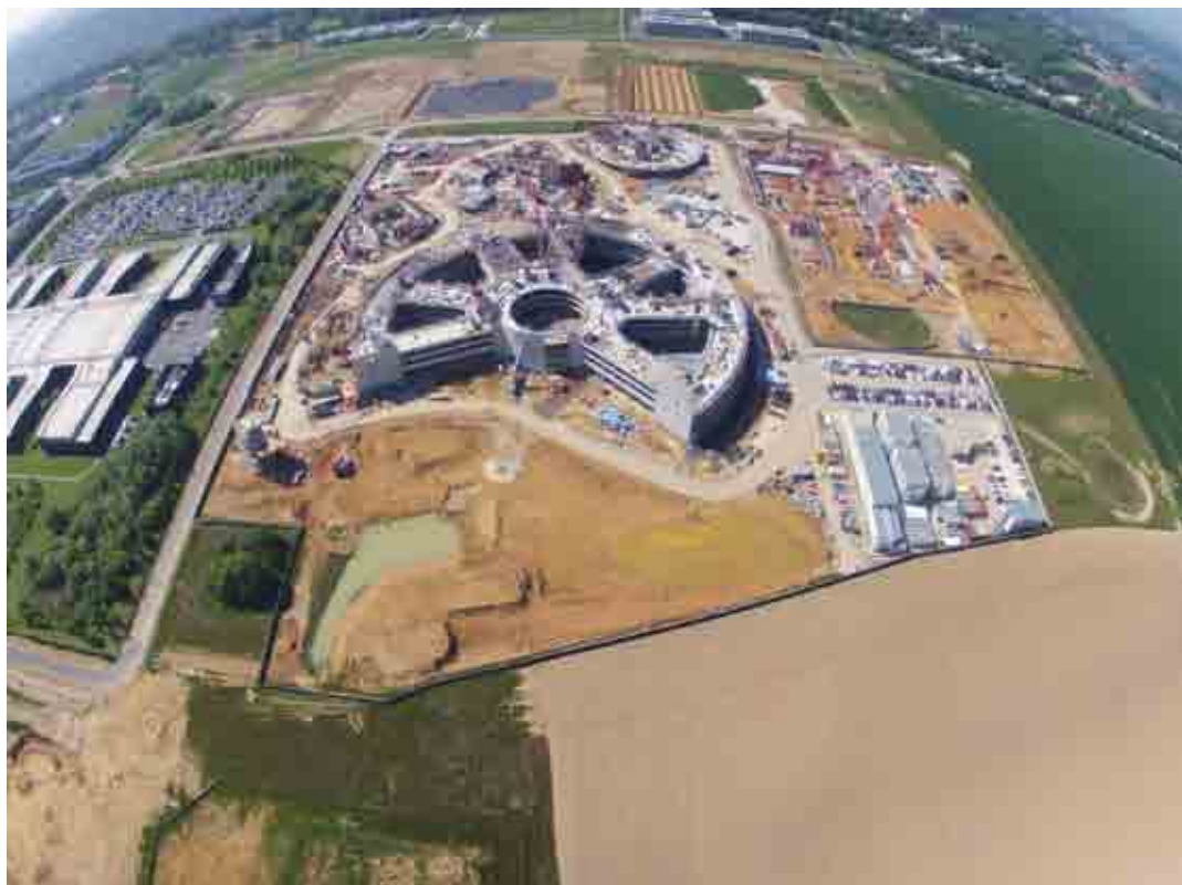
Photo-drone du chantier, mai, 2014 © Francis Soler Architecture
