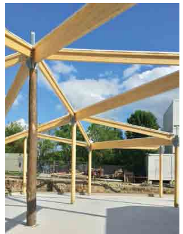
Chantier © Air Architecture
